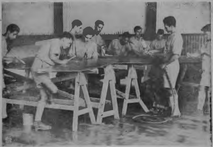
Engine Repair Workshop ( R.I.A.F. ) Fabric Workers Shop. ( R.I.A.F. )
